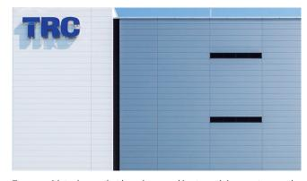
To cope with typhoons that have increased in strength in recent years, the wind load of exterior materials has been designed to be greater than the value specified by the Building Standards Law.
