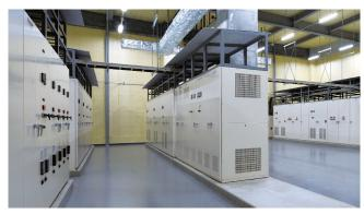
Considering flood/wind damage, an extra-high power substation is located on the 2nd floor of the building. A stable supply of large-capacity power is possible.
